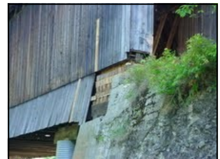
Siding repair area of Pier Bridge
